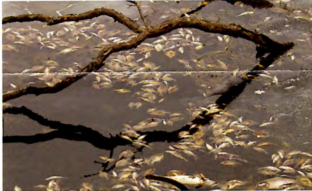
Dead fish downstream of the Beach O' Pines culvert - April, 2014
